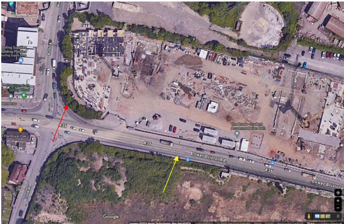
Figure 1 Satellite View of the Trial Site (Image ©googlemaps) with the SCOOT zone location arrowed yellow, controller location arrowed red.
