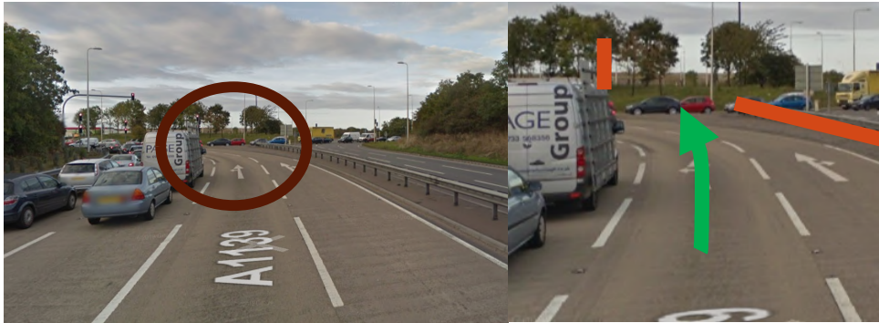
Figure 11. A1139 Junction 8, driver's centre of focus misses most of the signals (left) and the street furniture creates a misleading gap (right)
