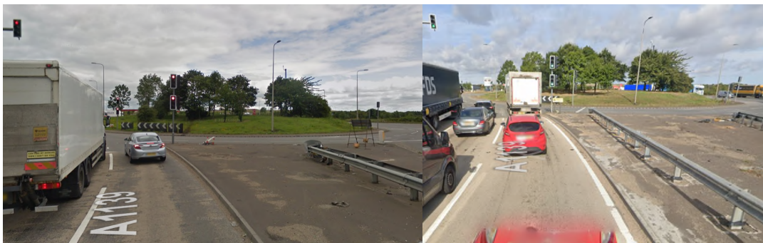
Figure 2. A1139 Junction 8 before (left) and after (right), Google Street View
