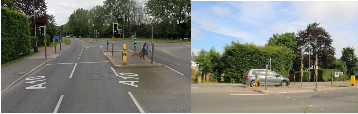
Figure 6. Approach to Harston Junction, Google (left), and a vehicle stopped having overshot the stop line, (right).
