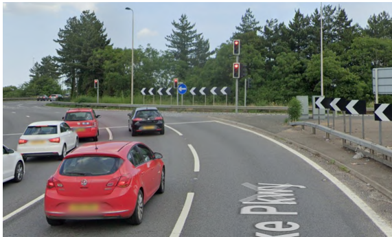
Figure 3. A47 Junction 20, designed with signals and clues to road alignment in the driver's line of sight, Google Street View
