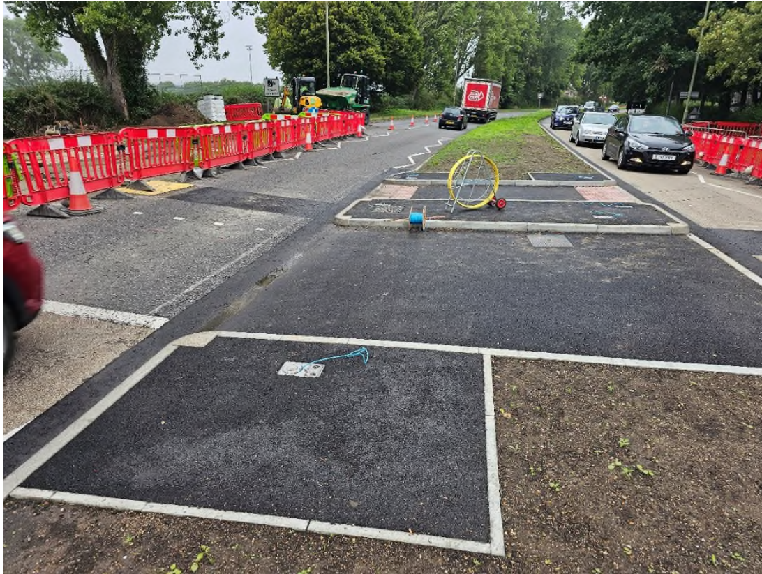
Figure 4 – Widened central island during construction
