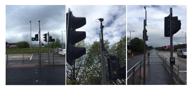
By configuring their position, size and function, each area activates a relay, triggered on movement of any vehicles or bicycles. The detection areas are also configured as presence detection zones, activating the relays until the point that the object leaves the zone. After several weeks in use, the council were satisfied that the radar detectors were operating successfully, day and night and in a range of weather conditions.
